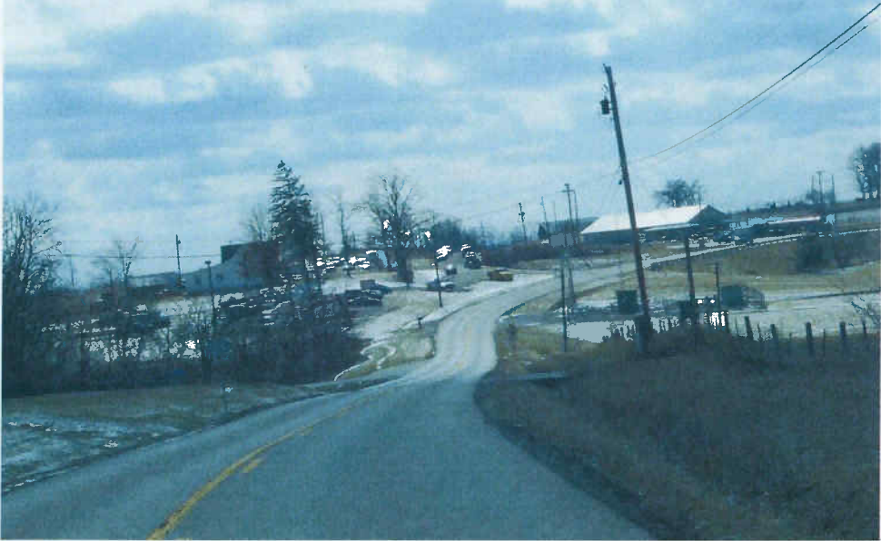
Looking East on KY 1448: Tom Browning Boys and Girls Club entrance on the left, entrance to a Columbia Gas substation on the right, and approaching the intersection of the AA.
