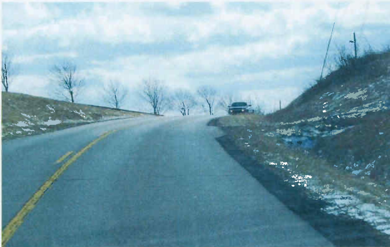
Horizontal - Vertical curve deficiencies located near the approach to the AA.
